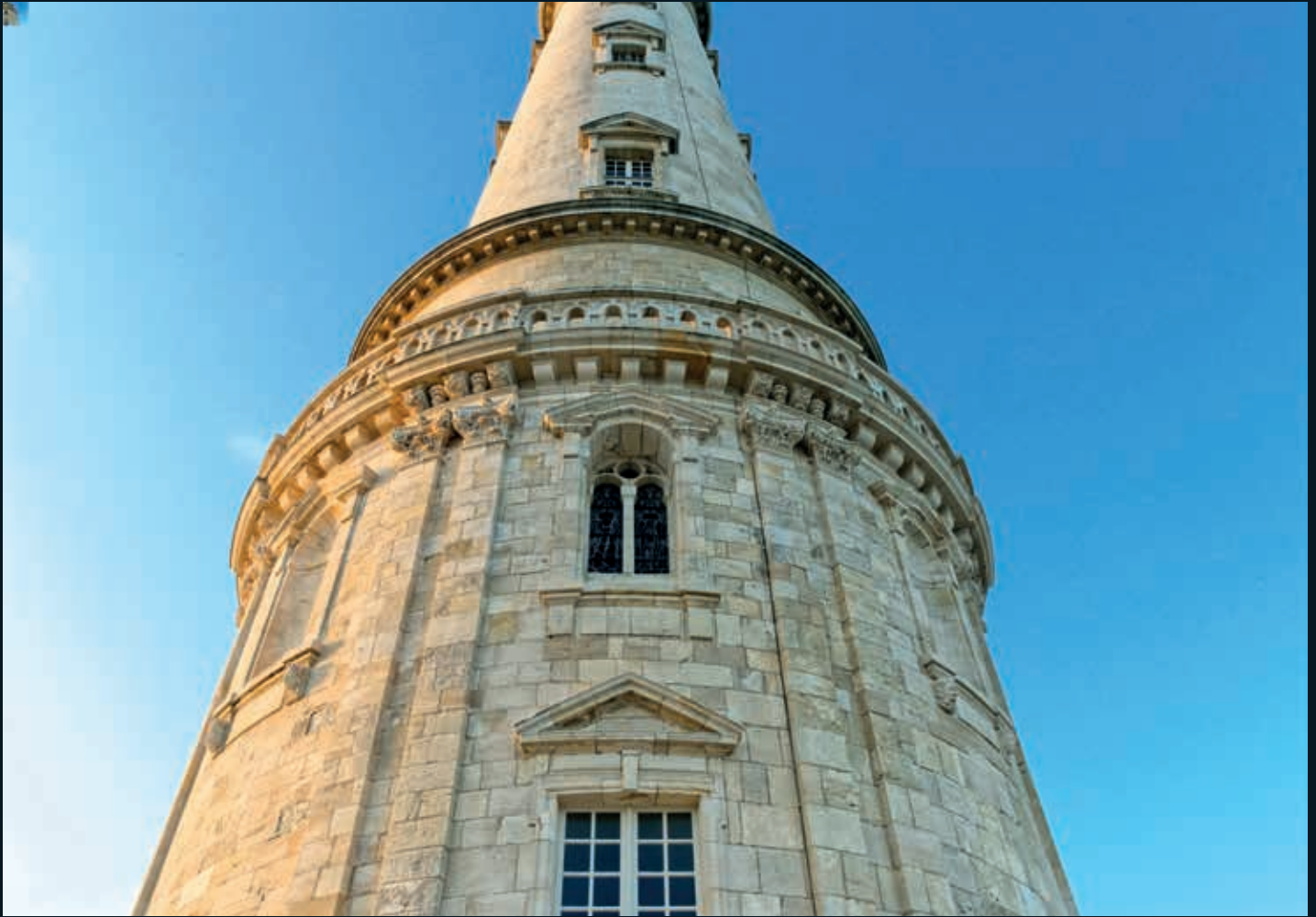
Cordouan Lighthouse (France).
