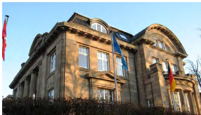
Building of the UNESCO Institute for Lifelong Learning (UIL) in Hamburg. © UIL
