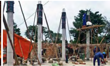
Construction of concrete poles
